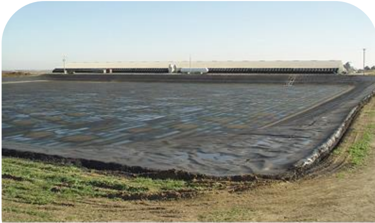
Figure 3. Geo-synthetic cover installed on a manure storage. Edge of the geo-membrane is typically trenched in. Note, these covers are not to be used as the storage should be surrounded by a fence.
